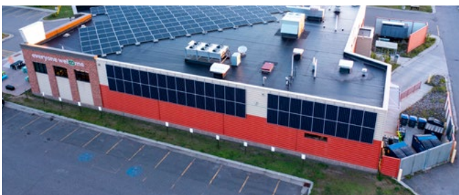
Southwest side solar panels were installed in 2016, during the construction of the Denfeld store.
